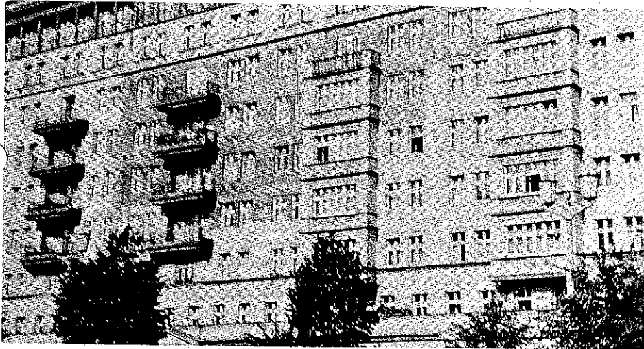
Here are buildings in pitiable condition along the former Stinallee (now Karl Marx Allee), the "showplace" of drab East Berlin. Nearly every one of the post-war constructed buildings has huge areas of exposed brick where the white tile overlay has fallen off.
